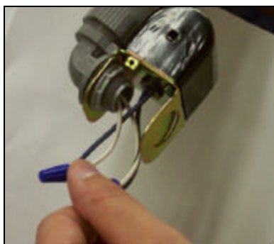
Straightening the wires
